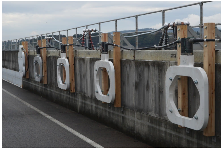
Fig. 6.28 Installation condition of test coils (from the back left, void A, shield exfoliation, void C, void B, abnormal connector)
