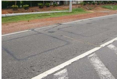
Figure 3.1(c) The WIM sensors in the road pavement
