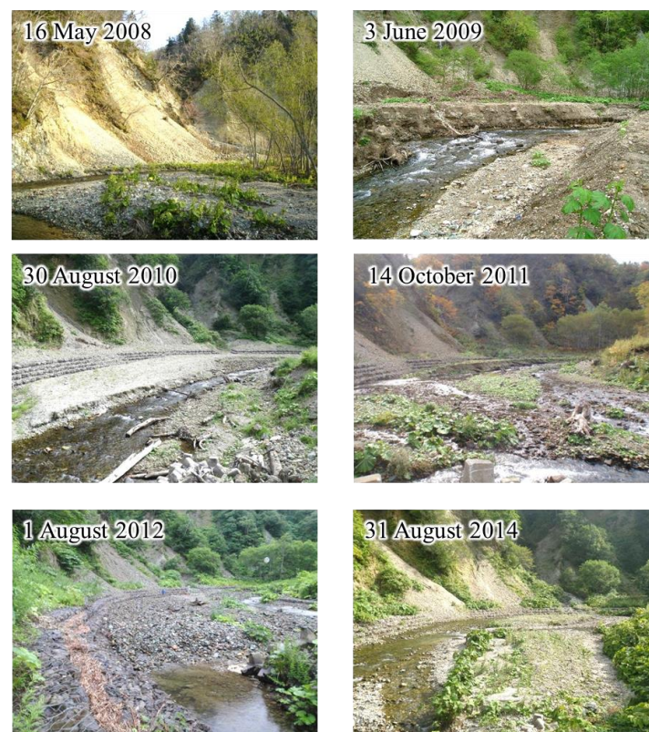
Figure A1. Upstream view from the check dam before (16 May 2008) and after (3 June 2009–31 August 2014) dam removal (February 2009). Before the removal, the check dam was filled with sediment. After the removal, the impounded sediment was eroded: initially, a narrow channel incised the impounded sediments, and then channel widening proceeded.
